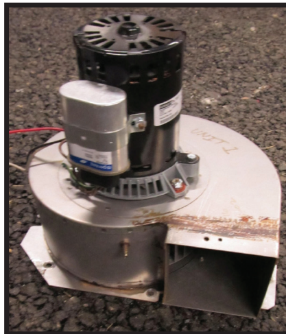
Figure 23. Venter Assembly (Refer to Table 35 )
