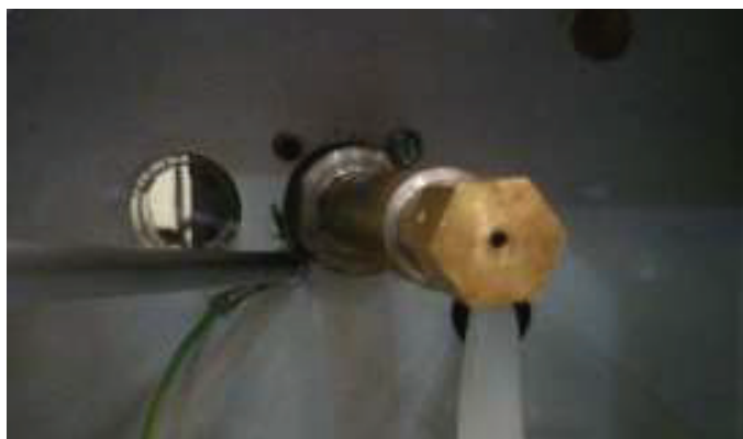
Figure 8. Gas Orifice Replacement for Unit Size 170 Models VCS, VCT, and VPT
