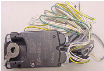
Figure 7. Inlet Damper Actuator
